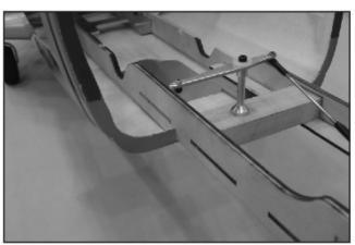
20. Remove the wood mount, then use file to make two notches so the wood rails can fit in later.
