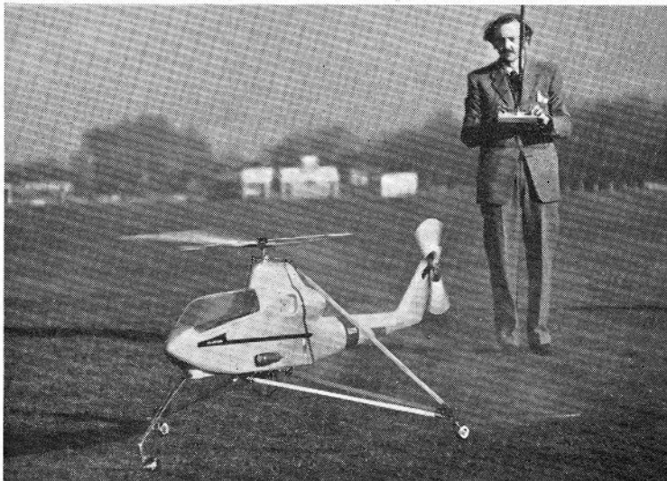
A modification to the training undercarriage is to fit castoring wheels. These are essential as, at first, one is never sure in which direction the model will skate off, or land, come to that, and fixed wheels would cause the 'copter to tip over more readily, which will break a rotor blade or, at the very least, bend the blade mounting plates and the stabilizer blade rod, necessitating a return to the workshop for repairs and re-alignment. Standard steerable nosegear is easily modified, as shown right.
